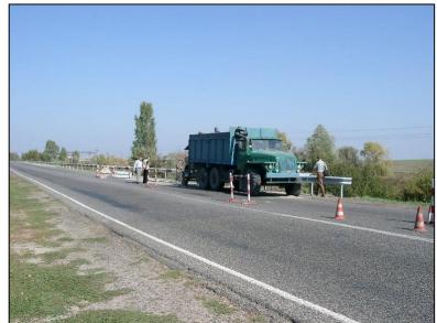
For the surface preparation, a mobile URAL truck-mounted sandblasting unit was used. After sandblasting the old hot-dipped crash barriers, the average surface roughness was Rz 15  $\mu$ m. The DFT of airless sprayed ZINGA was 90  $\mu$ m.
