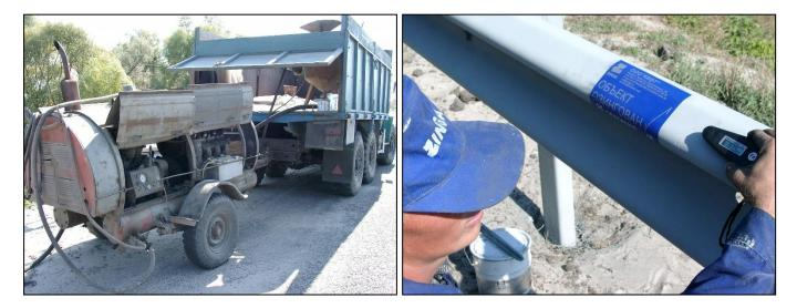
All the crash barriers protected with **ZINGA**, imported and marketed by **Vector Technologies Co.**, are marked with special durable stickers containing the date of application (here: 20th September 2003) and **Vector Technologies Ltd.** contact data. System: Surface preparation: Sandblasting Rz 15 μm ZINGA (airless spray): 90 μm DFT
