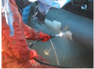
System: Surface preparation: Wet blasting and machine cleaning to ST3 ZINGA 1 x 80 µm DFT (by brush & roller) ZINGALUFER 1 x 40 µm DFT Local topcoat 2 x 40 µm DFT
