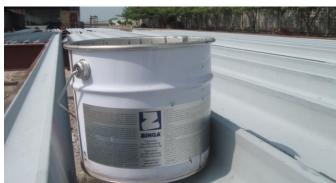
System: Surface preparation : Blasting to SA 2.5 and Rz 50-70  $\mu$ m ZINGA 2 x 60  $\mu$ m DFT
