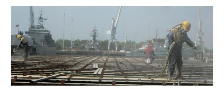
These tracks at the **Navy Dockyard** were protected against heavy corrosion (caused by the location of the tracks in the splashzone) with a **ZINGA** unique system.
