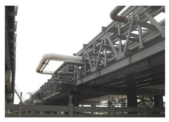
In 2009, **ZINGA** was used to repair rust spots on the jetty (gas pipes and supporting structure). Up till today around 15,000m<sup>2</sup> of the 50,000m<sup>2</sup> structure has been repaired using **ZINGA** and **ZINGALUFER**.
