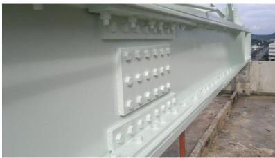
System: Surface preparation: Wet blasting ZINGA 1 x 80 μm DFT (by brush & roller) ZINGALUFER 1 x 80μm DFT Local topcoat
