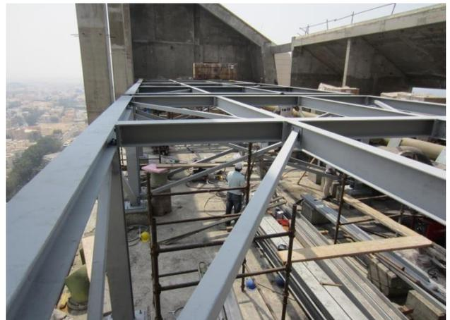
During construction of the building from 2010 until 2013, **ZINGA** was specified instead of hot dip galvanization (by **Saudi Diyar Consultant**) for about 30 tons steel beams at the water treatment station located at an open area on the 16th floor of the Eastern tower.
