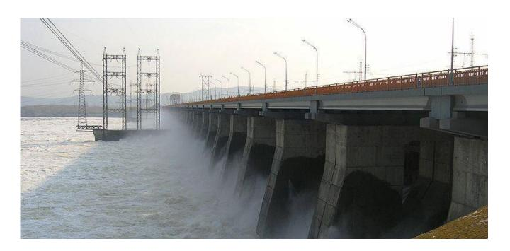
In 2011 maintenance began on flow regulating valves of the spill over. After cleaning and roughening of the surface, **ZINGA** was applied by spraying with a layer thickness of 100  $\mu$ m DFT.
