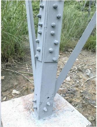
Surface preparation: Thorough decontamination of old hot-dip System: ZINGA 1 x 60µm DFT
