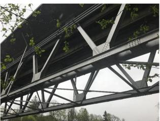
Photos are from May 2016, after 15 years of exposure. The system is still intact without any sign of brakedown or
