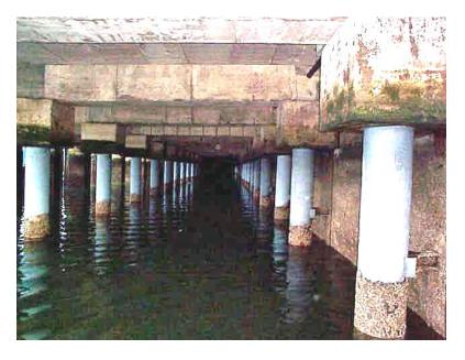
**ZINGA** was applied on immersed piles of a pier in the Bangor harbour. The piles were first UHP water-blasted and then gritblasted to give the correct surface profile. Then approx. 200 μm of **ZINGA** was applied in 4 coats by brush. The work was executed by the contracting company **SAR Marine and General** in November 2000.
