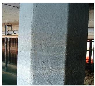
These pictures of the pier legs were taken in August 2001: one year after the application. The **ZINGA** is holding perfectly with no rust showing. Any marking on the legs is either seaweed or harbour contaminants.
