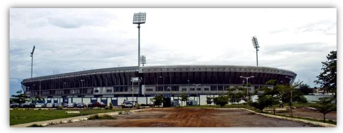
The light mast structures are hot-dip galvanized structures with a height of 48 meters and a base perimeter of 4,5 meters, erected on a secured concrete base. The four light masts, have an existing hot-dip galvanized layer with serious corrosion, on the mast head-frame assembly, the upper platform assembly and flooring, mast base plate and some areas of the main mast shaft.
