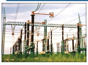
The pylons and other structures of the **Krasikov Transformer Station** were protected with **ZINGA** in the summer of 1994. The application was done by brush and roller. **ZINGA** was used as primer on the grit-blasted surface in one layer of approx. 50  $\mu$ m. The total amount of **ZINGA** used at this site was approx. 1.5 ton. **ZINGA** was topcoated with Jotun Conceal (without sealer) at a layer thickness of 80  $\mu$ m applied in one coat, also by brush and roll.
