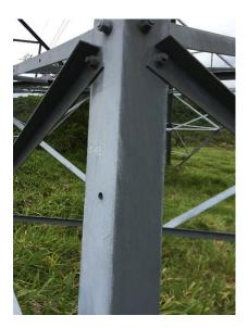
To date, **ICE** still uses **ZINGA** to maintain its power pylons and transmission antennas.
