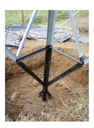
In 2009 they conducted a test with **ZINGA** as unique system for the above-ground parts and with a **ZINGA + ZINGATARFREE** system for the underground parts.
