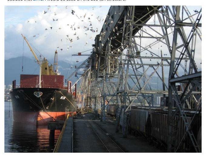
**ZINGA** was used on all the larger - non-mobile - parts of the structure.
