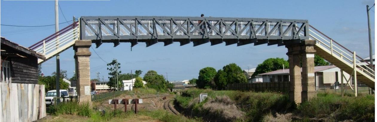
The below Queensland Rail Bridge was protected with **ZINGA** on 26-06-2003. The bridge identification number 902-788 was coated according to **Queensland Rails specification**. On June 20, 2007, an inspection was performed.
